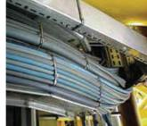
Manufactured in the UK from 316 SS, the selectively coated Ball-Lok ties offer the same benefits as the full coated version but is ideal where Nylon 11 coating is required.
